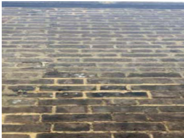
Existing cementitious mortar and brickwork damage to the west elevation of the listed building
